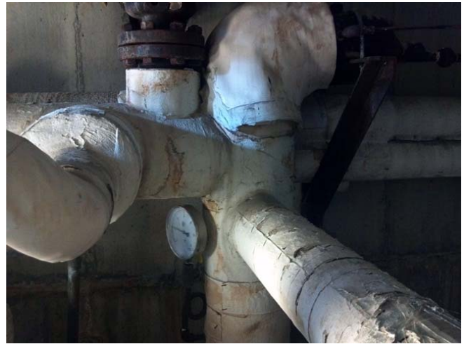
Pipe Insulation – Fittings, Elbows, Mudded Joint Packing (Photo 02)
