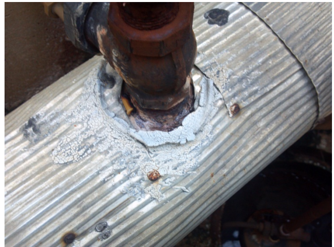
Caulking/Putty Located on Pipe Wrap (Photo 04)
