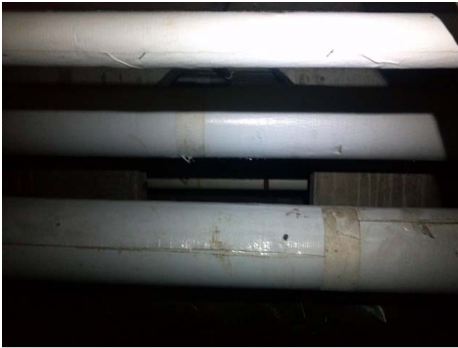
Mastic Coating on Thermal Pipe Insulation (Photo 01)
